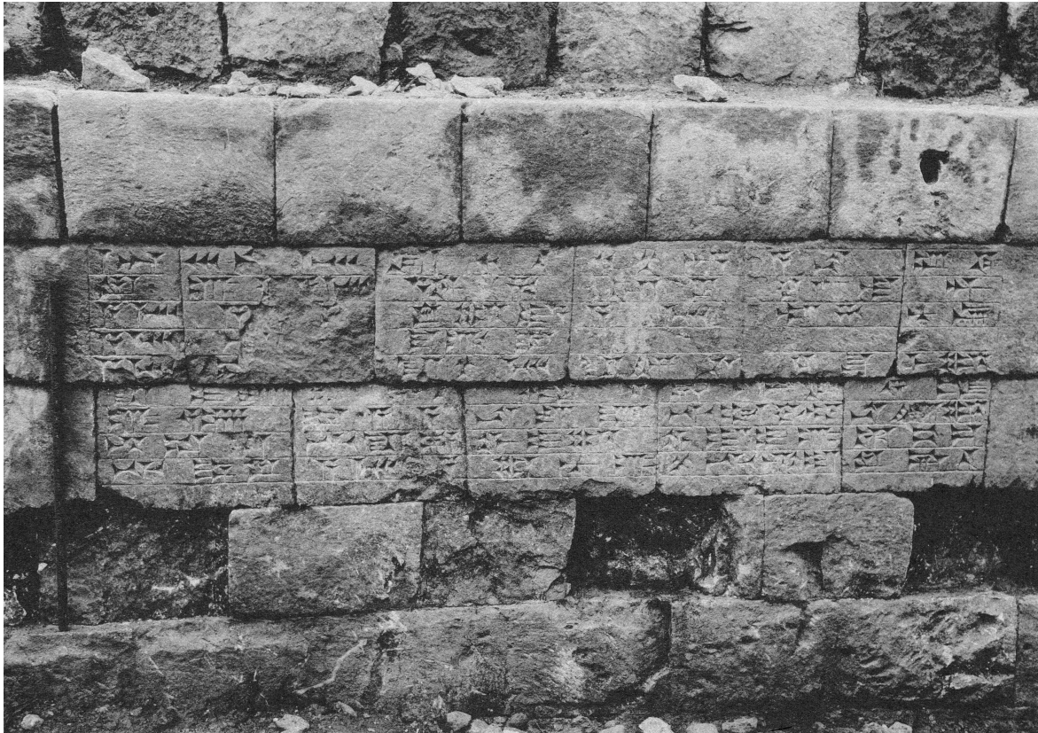
Figure 26. One set of stone blocks (text no. 226) found on the sixth bay of the aqueduct at Jerwan recording the construction of an aqueduct. Reprinted from Jacobsen and Lloyd, OIP 24 pl. XVI C courtesy of the Oriental Institute of the University of Chicago.
