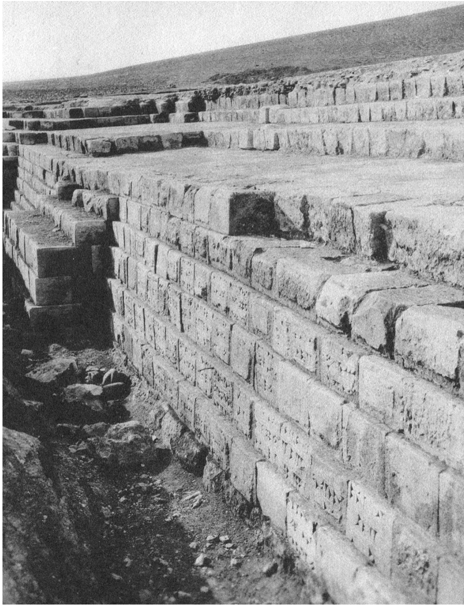
Figure 29. A section (no. 1 on fig. 28) of the south façade of the Jerwan aqueduct with reused stone blocks inscribed with text no. 228. Reprinted from Jacobsen and Lloyd, OIP 24 pl. X A courtesy of the Oriental Institute of the University of Chicago.
